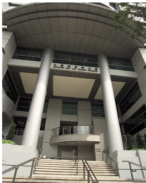
新九龍城裁判法院大樓正門入口處 The main entrance of the new Kowloon City Law Courts Building
